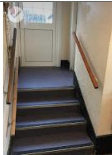
Access to the female toilets is stepped. Turning is limited at head of the stairs.
